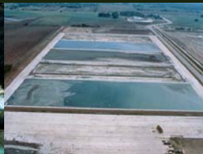
25 acre sludge drying basins in Austin, TX
