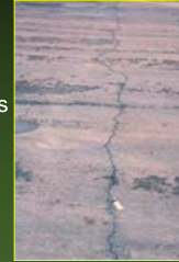
New, Unsealed Crack
