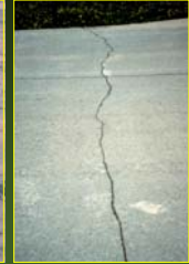
10-yr Old Sealed Crack
