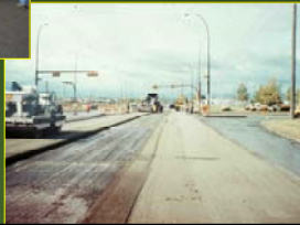
Intersection Replacement Calgary, AB
