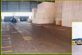
Interior Floor Lynnterm Terminal Port of Vancouver, BC
