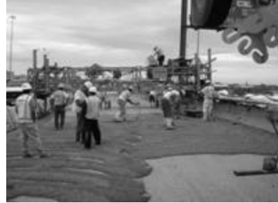
Concrete mix at time of placement.
