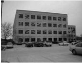
Illinois DOT, District 1 parking lot, 45,000 sqft. 2" thick, 7.5 lbs/cy Example Macro Fiber, joints at 24" 4" thick, 4 lbs/cy Example Macro Fiber, joints at 48"
