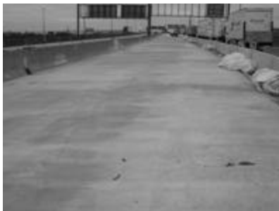
Finished overlay after wet cure
