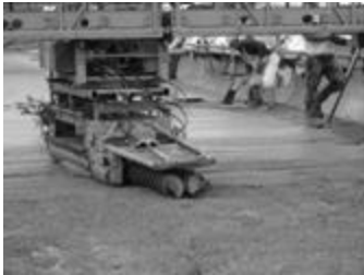
Spreading concrete
